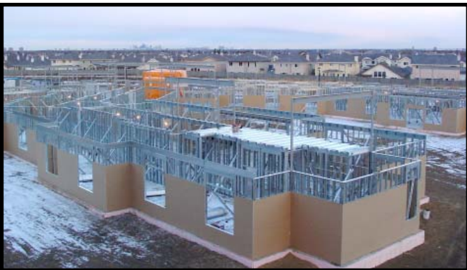
Construction on the Health Services Neighborhood at Touchmark.
